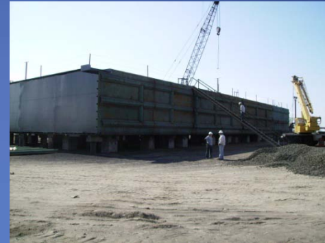
Barge construction progress survey
