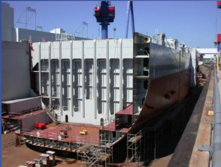
Container ship construction progress survey
